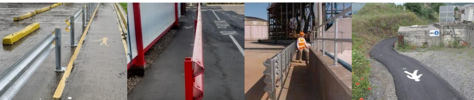
Examples of physical barriers and a separated walkway
