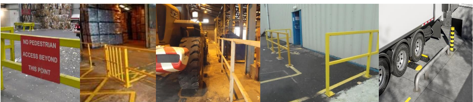
Examples traffic barriers/fencing inside MRF buildings, example pedestrian barrier just outside an access door, and an example lorry 'bump stop' to prevent the vehicle's rear overhang impacting a building
