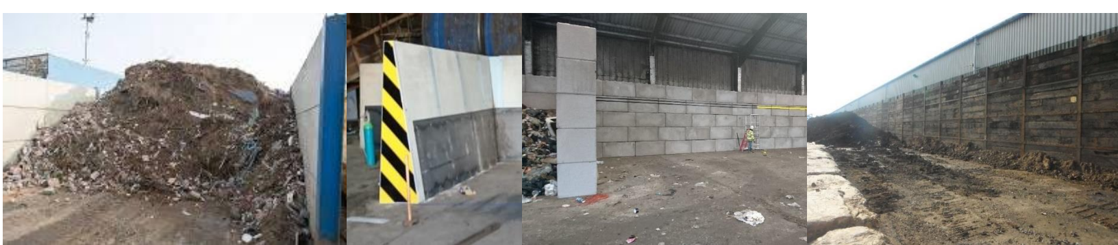
Typical examples of some of the types of containment walls used at waste and recycling sites
