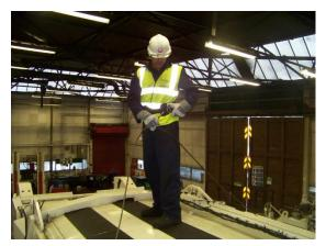
Fall arrest /restraint systems: Bi –Lines and fall arrest systems are suitable in particular for maintenance work required on the roof of the body of a vehicle and should be fitted to any to any vehicle where working at, and/or falling from, height during operation or maintenance presents significant risk.
